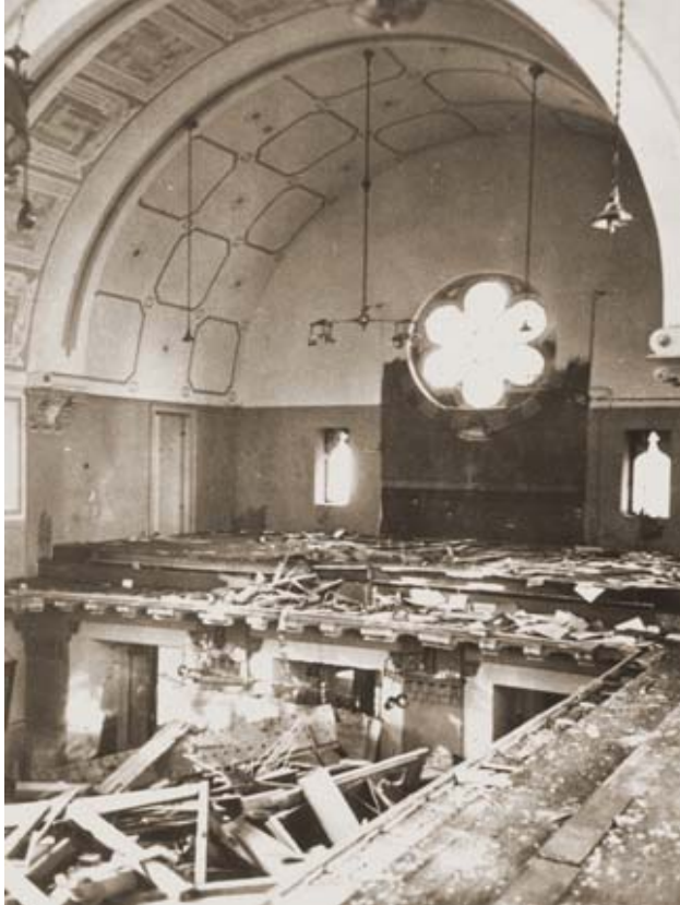
Destroyed Zerrennerstrasse synagogue – USHMM photo 97574
